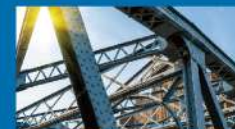
steel structure construction
